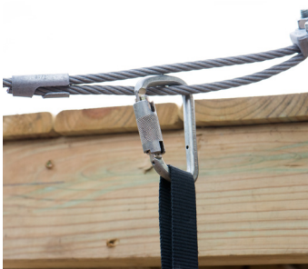
✗ Dead End of Cable with Serving Sleeve
